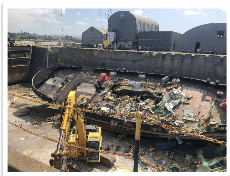
"Black Kite" Demolition at Dry Dock, Mare Island
