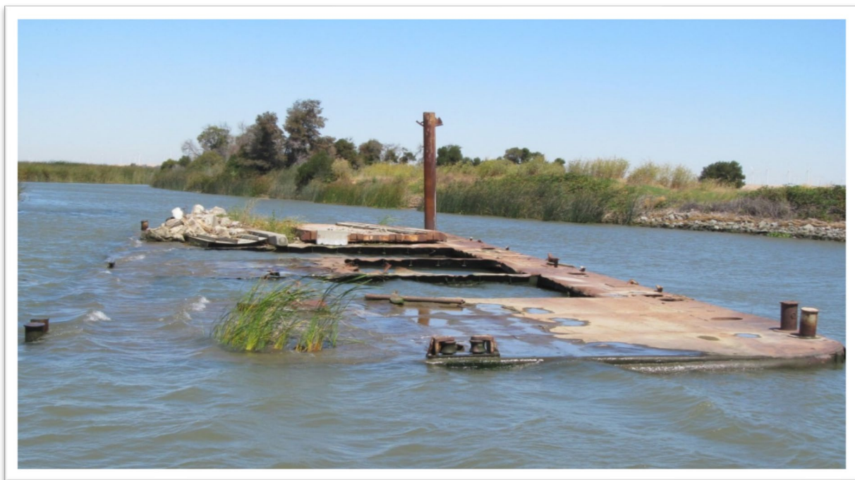
Sunk & Abandoned Spud Barge, New York Slough
