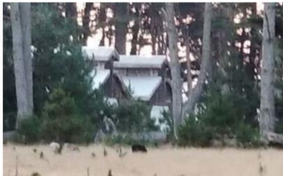
Private Cable Landing Station
