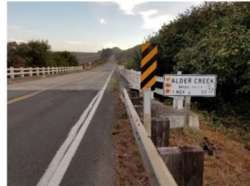
Alder Creek Bridge, conduit will either be attached to bridge or drilled below the creek, facing north
