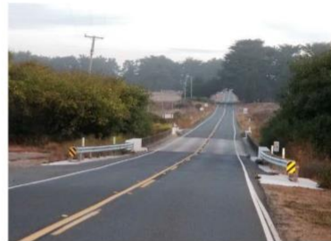
Brush Creek Bridge, conduit will either be attached to bridge or drilled below the creek, facing north
