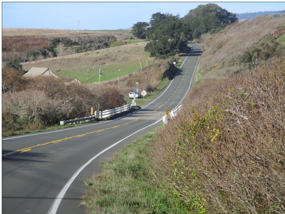
Photo 6. Facing north toward Alder Creek, view of State Route 1 segment where fiber cable may be installed within the roadway.
