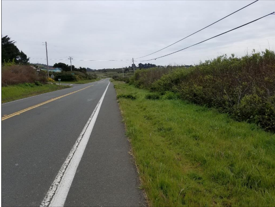
Photo 7. Facing south, representative view of the non-native annual grass adjacent to State Route 1 where underground conduit installation would occur. Classified as an environmentally sensitive habitat area, the sensitive natural community coastal dune willow thicket is adjacent to the non-native annual grassland.
