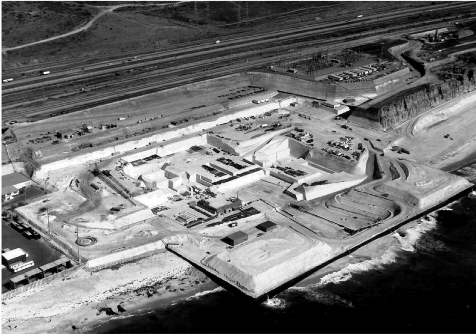
SITE CONSTRUCTION AERIAL PHOTO (ca. 1970s)
