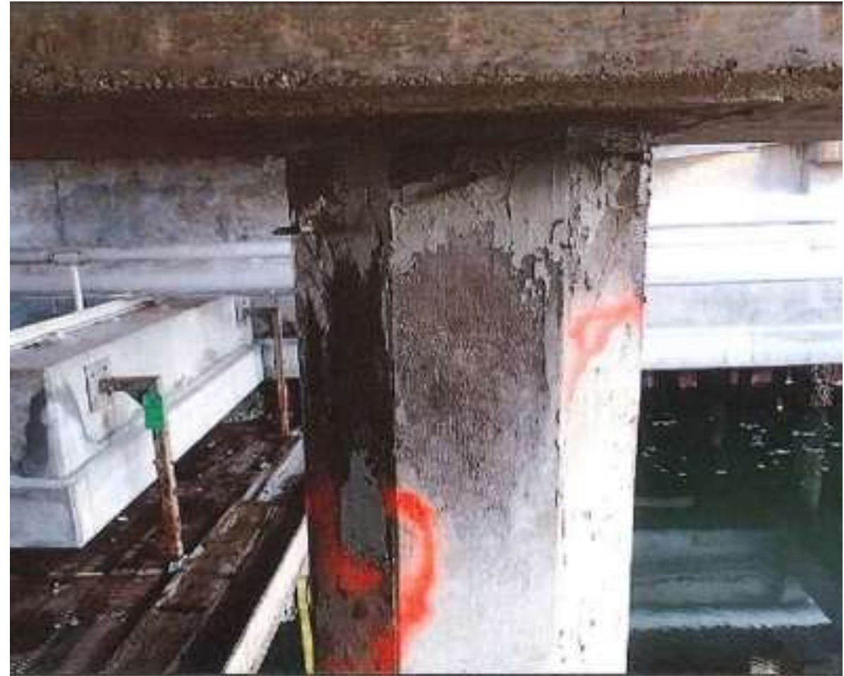
Pile Epoxy Injection Repair
