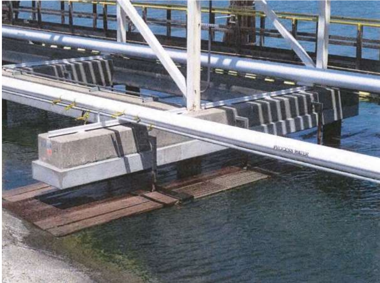
Beam Full Soffit Repair
