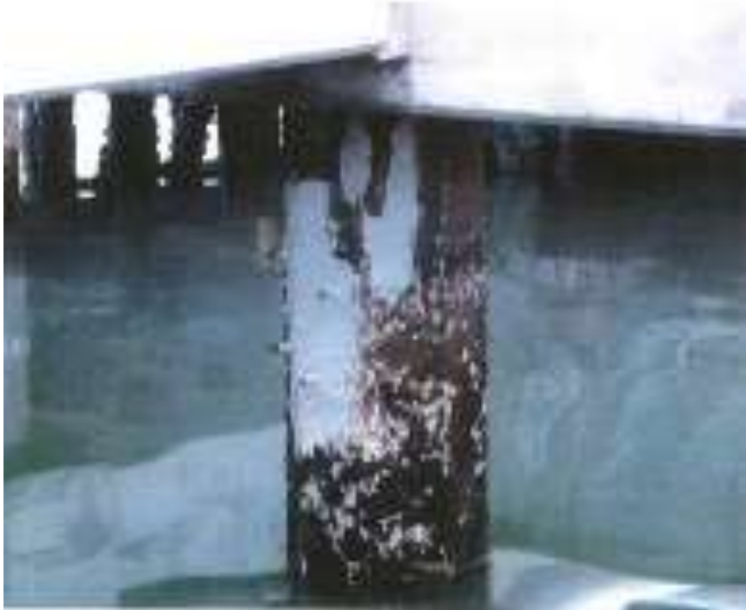
Pile Epoxy Injection Repair
