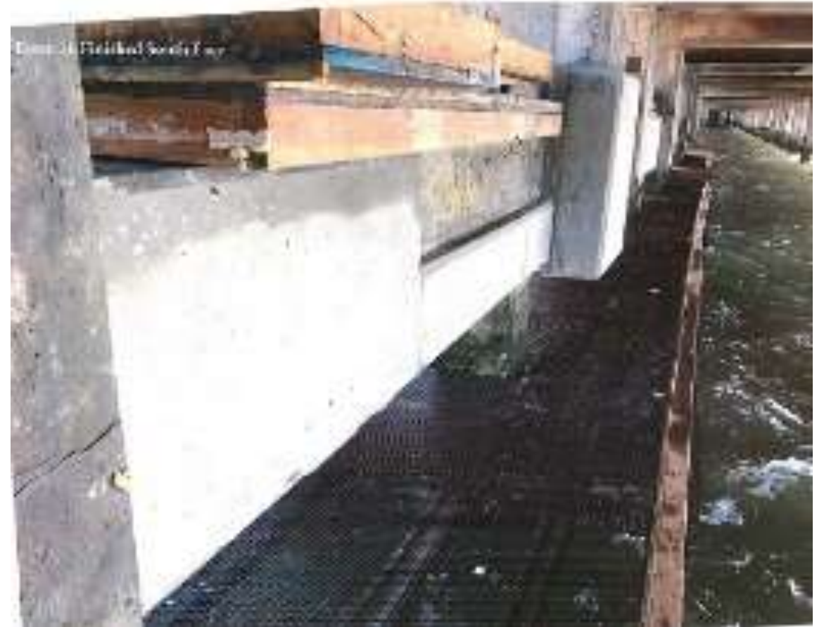
Beam and Column Repair
