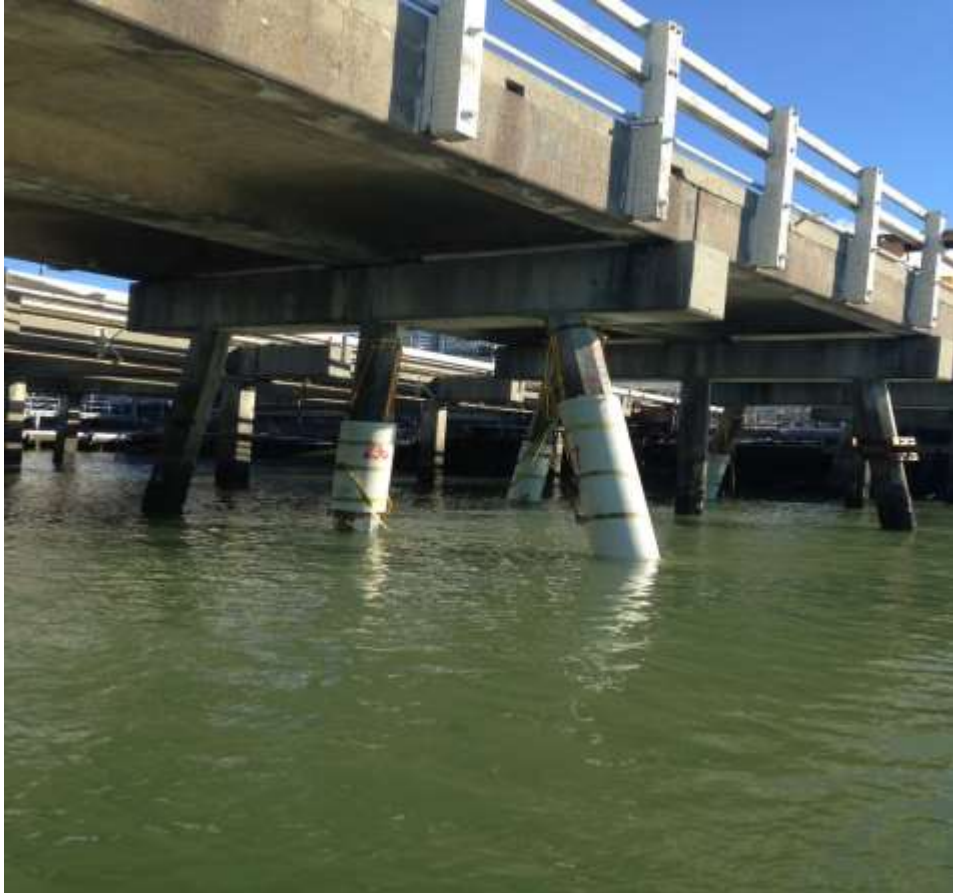
Pile Grouted Sleeve Repair
