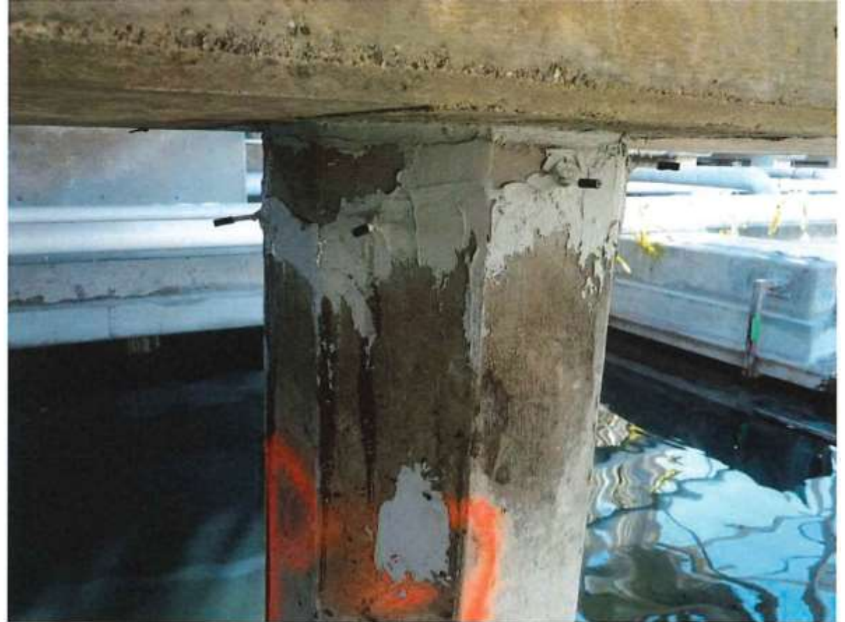
Pile Epoxy Injection Repair
