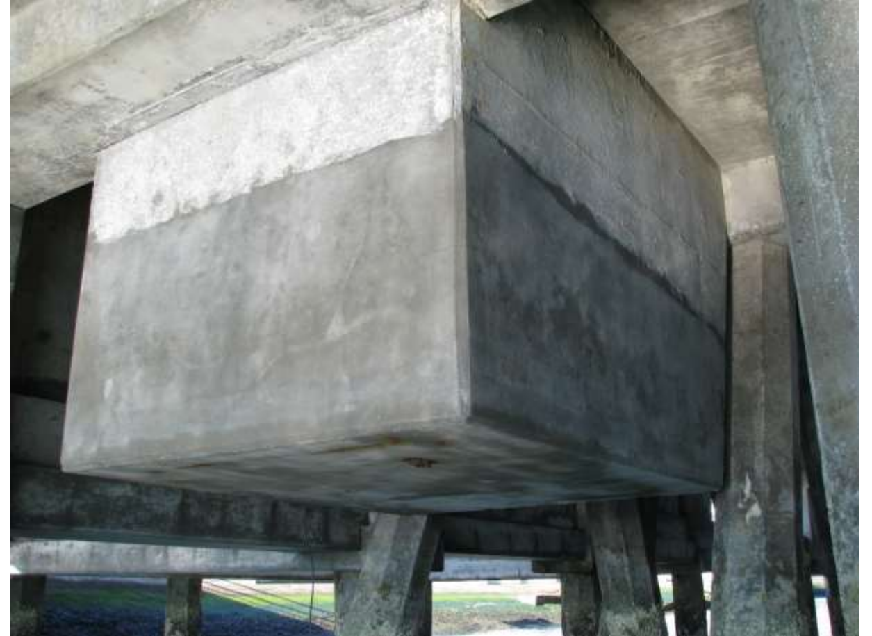
Utility Vault Repair
