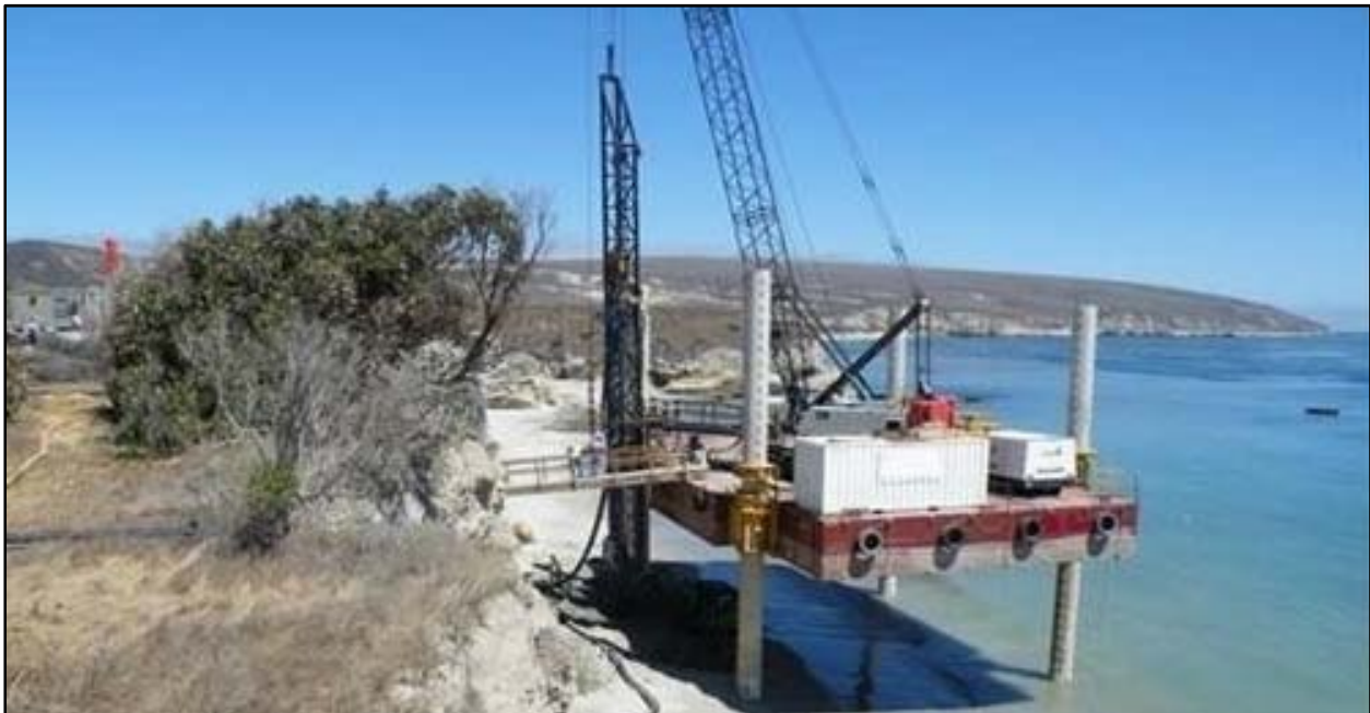
Figure ES-3. Typical Jack-up Barge Configuration in Nearshore Setting
