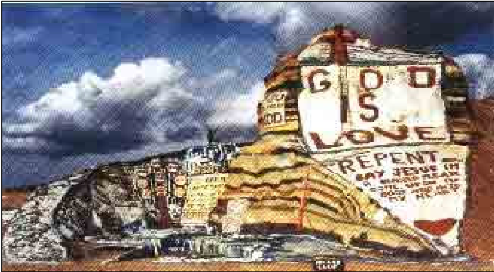
Figure 7: First Salvation Mountain before it collapsed in 1990 (www.salvationmountain.us, 2004).
