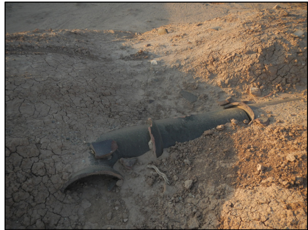
Figure 20: EDS-05, 12" diameter sewer pipes exposed by erosion.
