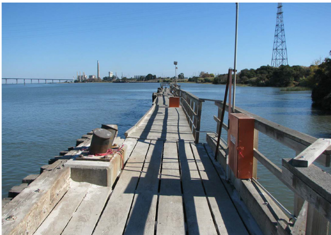
Dolphin G & Walkway Deck (to be demolished)
