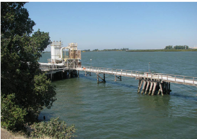
Dolphin G & Walkway Deck (to be demolished)
