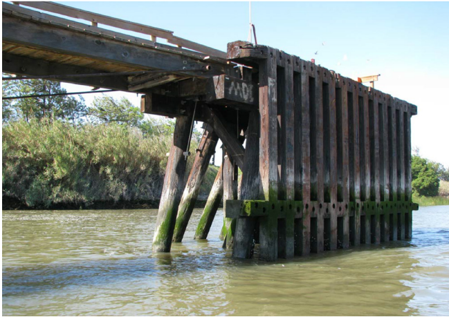
Dolphin A (to be demolished)
