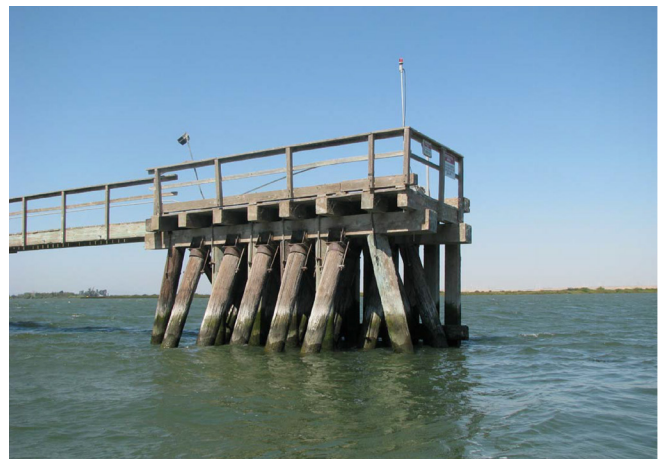
Dolphin I Framing and Piles (to be demolished)
