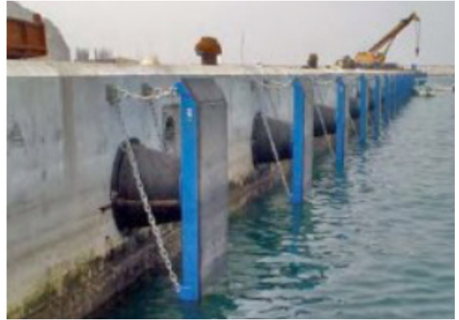
Dolphins with Fender Systems
