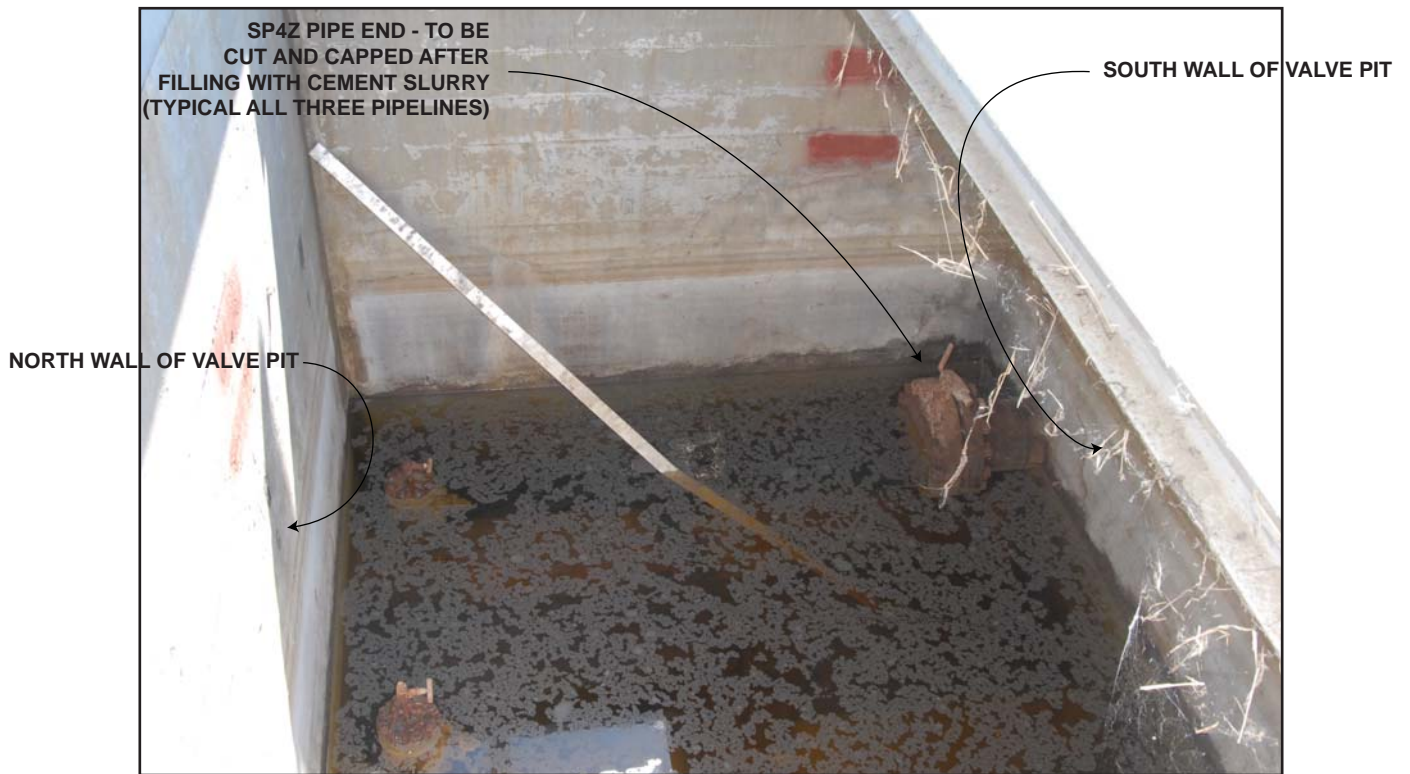
PHOTO 2 - INTERIOR OF SOUTH LANDING VALVE PIT
