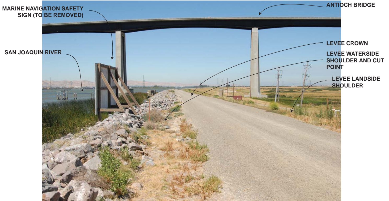
PHOTO 1 - SHERMAN ISLAND LEVEE AT NORTH LANDING.
