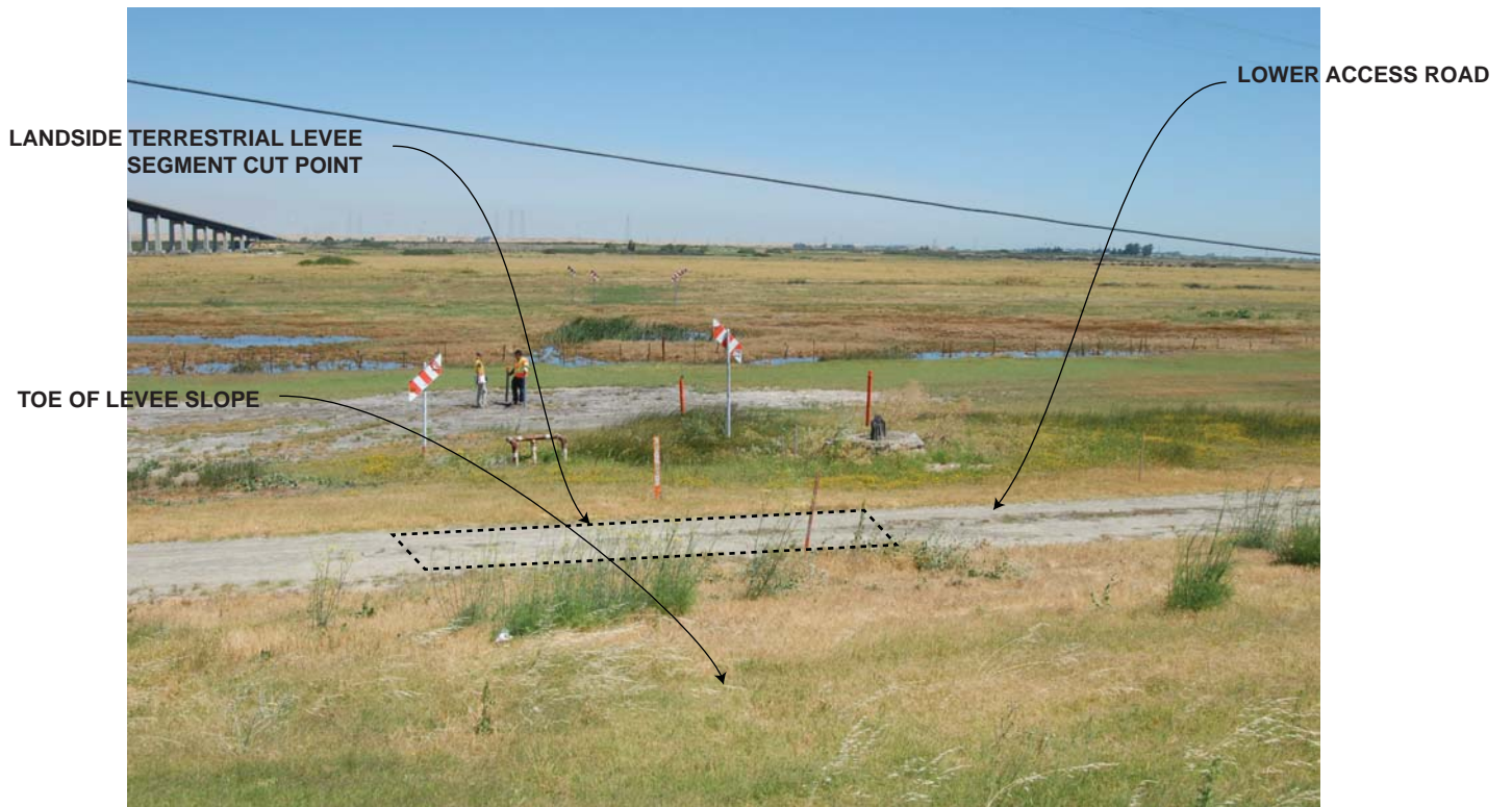
PHOTO 4 - LANDSIDE TERRESTRIAL LEVEE SEGMENT CUT POINT
