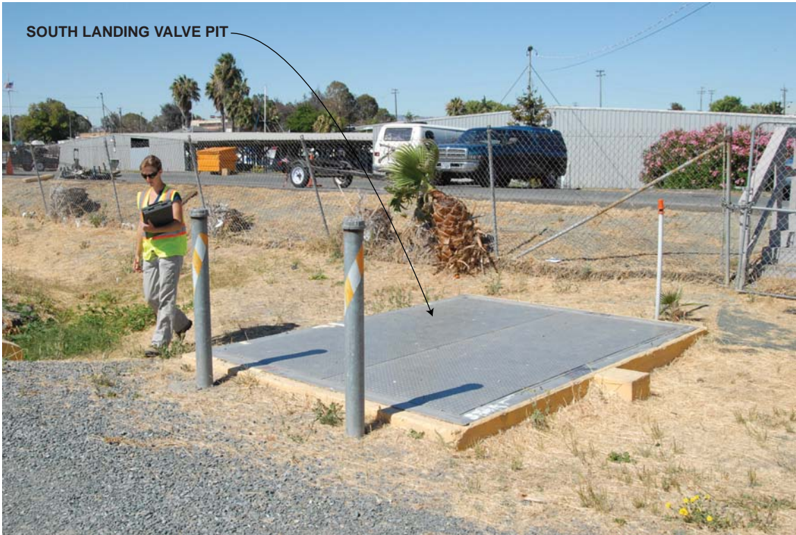
PHOTO 1 - SOUTH LANDING VALVE PIT - INSIDE LAURITZEN YACHT HARBOR
