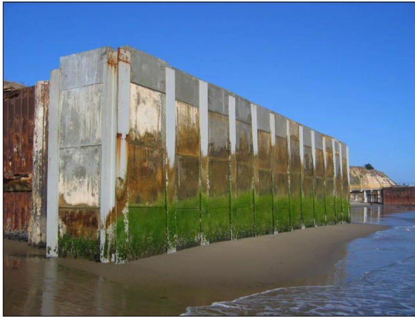
Figure 4.2-3a Pier 421-1 Caisson Wall (facing ocean)
