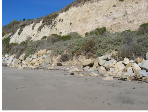
The existing aging timber bulkhead seawall has been reinforced through much of its length with a rip-rap boulder revetment, although some gaps in this protection exist.
