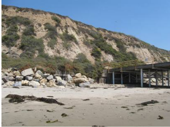
The Project's existing timber and rock seawall appears generally intact along most of its reach, although the eastern end (outside of critical pipeline areas) has suffered some wave damage.
