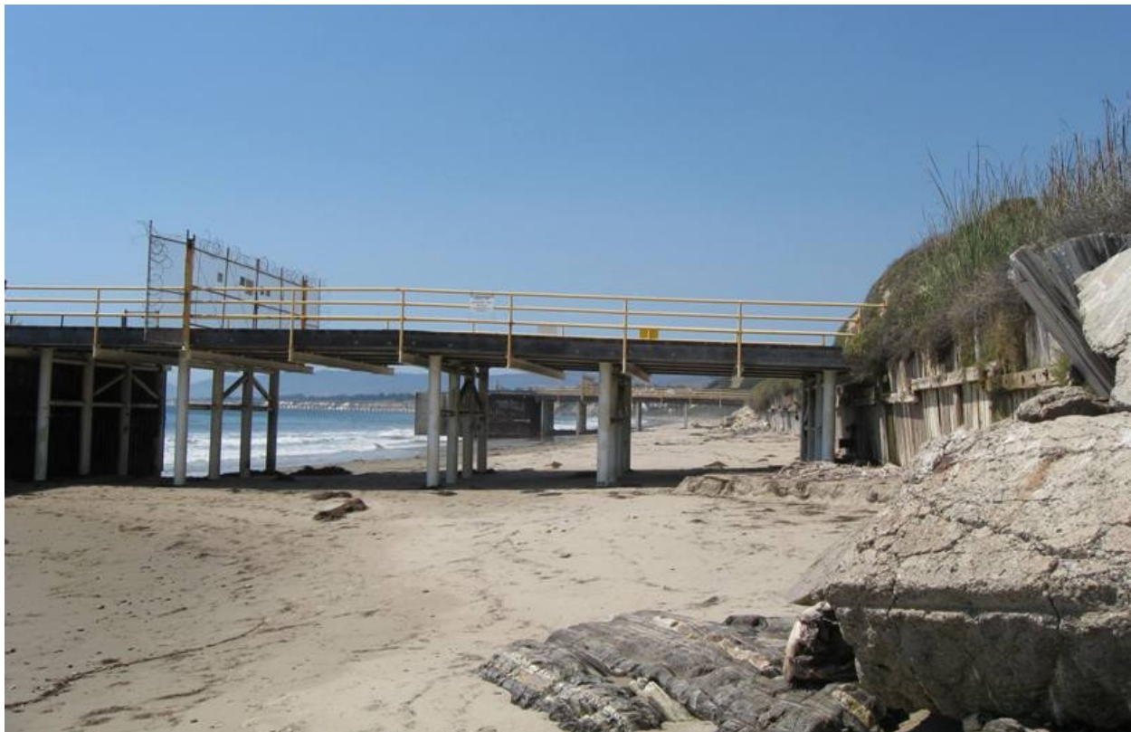
FIGURE 4.12-1. CURRENT VIEW OF PIER 421-2 FROM THE BEACH SHOWING PEDESTRIAN BEACH ACCESS
