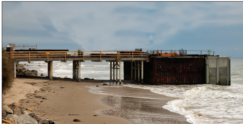
Figure 4.2-2b Pier 421-2 (shown under repair as of April 2011) (Photo: Bruce Reitherman)
