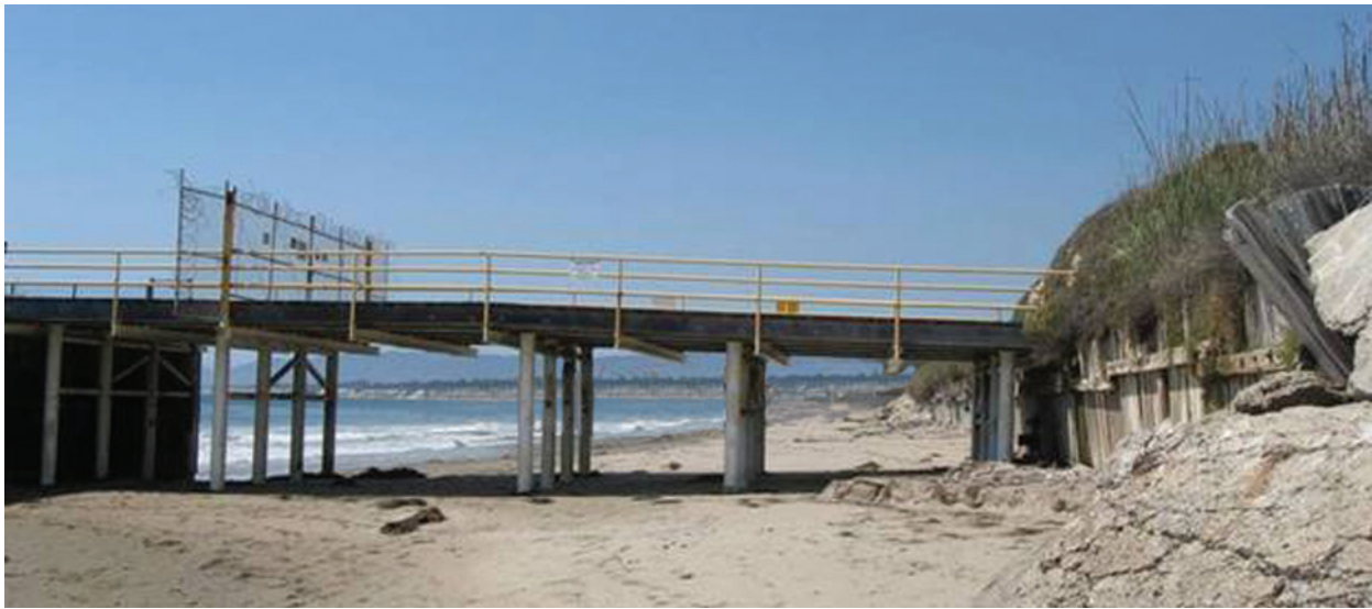
14 FIGURE 4.12-3. VIEW OF PIER 421-2 FROM THE BEACH WITH REMOVAL OF 15 PIER 421-1
