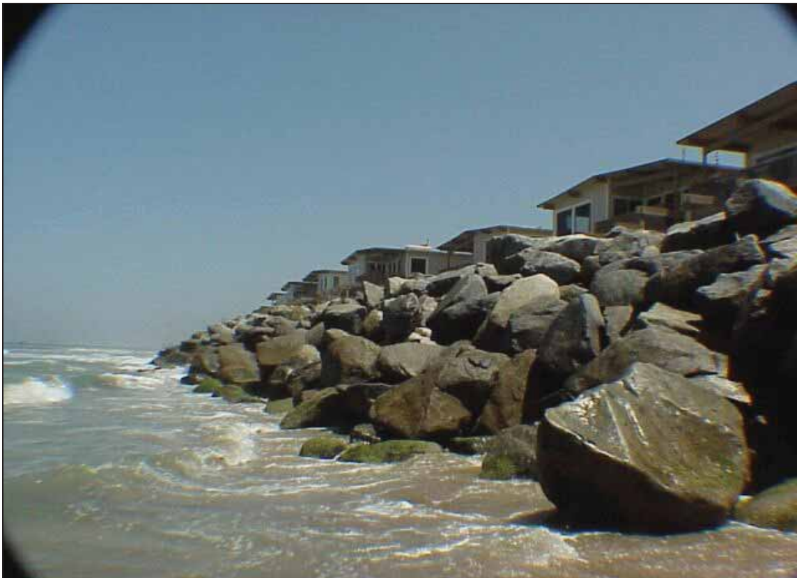
Figure 7. Armor Stone Revetment at San Clemente, California, USA.
