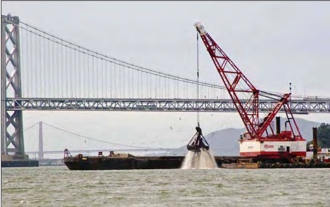
Figure 4. Maintenance Dredging in San Francisco Bay, California, USA.
