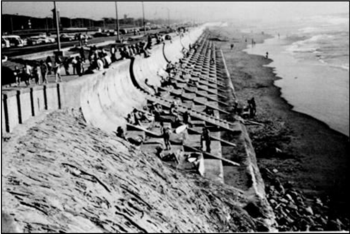
Figure 6. O'Shaughnessy Seawall at the Great Highway, San Francisco, California, USA.
