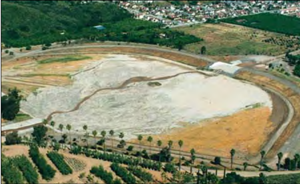
Figure 5. Debris Basin in Riverside, California, USA.
