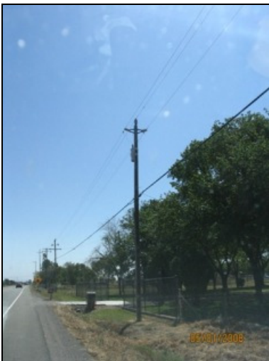
Photo 78: A pole mounted transformer located in the subject corridor.
