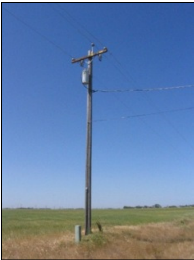
Photo 86: A pole mounted transformer located in the subject corridor.
