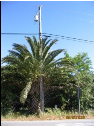
Photo 68: A pole mounted transformer located in the subject corridor.
