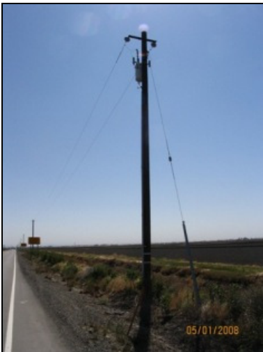
Photo 63: A pole mounted transformer located in the subject corridor.
