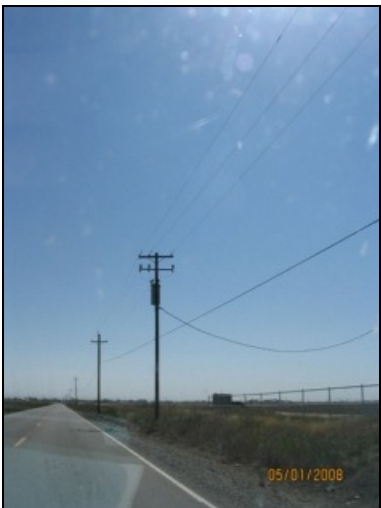
Photo 66: A pole mounted transformer located in the subject corridor.
