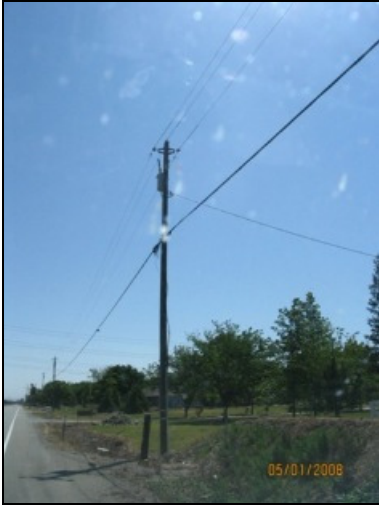
Photo 76: A pole mounted transformer located in the subject corridor.
