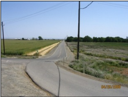
Photo 62: The subject corridor viewing in a northerly direction.
