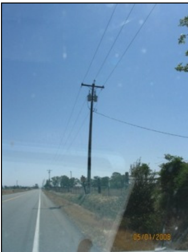
Photo 81: A pole mounted transformer located in the subject corridor.
