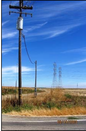
Photo 13: A pole-mounted transformer on the southeast corner of Option E viewing in a northerly direction.
