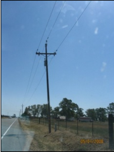
Photo 82: A pole mounted transformer located in the subject corridor.
