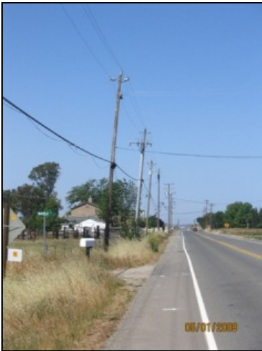
Photo 74: A pole mounted transformer located in the subject corridor.
