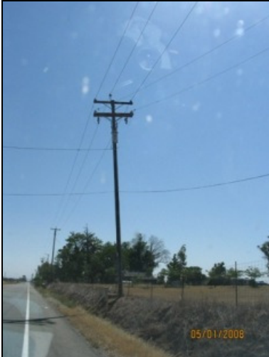
Photo 79: A pole mounted transformer located in the subject corridor.
