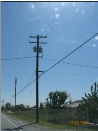
Photo 72: A pole mounted transformer located in the subject corridor.
