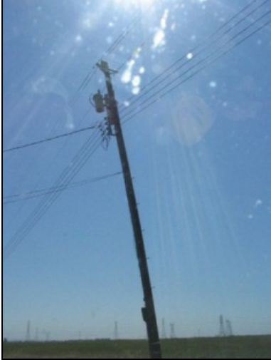
Photo 85: A pole mounted transformer located in the subject corridor.
