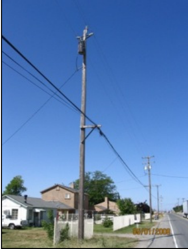
Photo 73: A pole mounted transformer located in the subject corridor.
