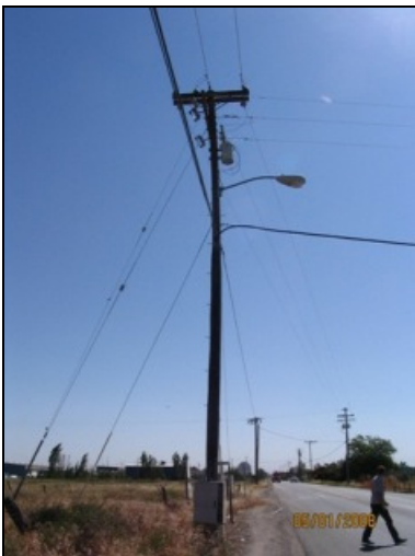
Photo 69: A pole mounted transformer located in the subject corridor.
