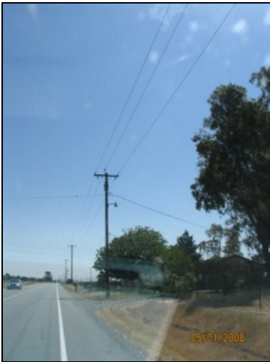
Photo 83: A pole mounted transformer located in the subject corridor.
