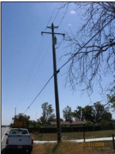
Photo 75: A pole mounted transformer located in the subject corridor.
