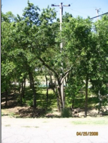
Photo 61: A pole mounted transformer located in the subject corridor.
