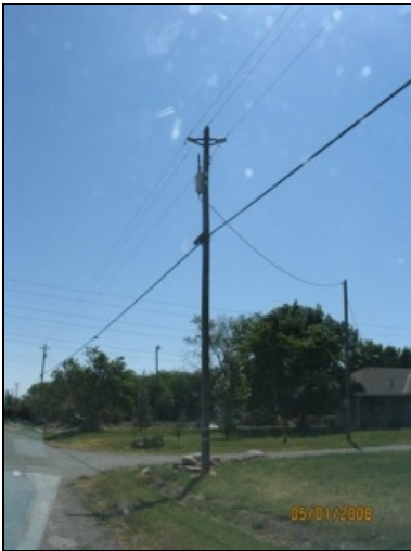
Photo 77: A pole mounted transformer located in the subject corridor.
