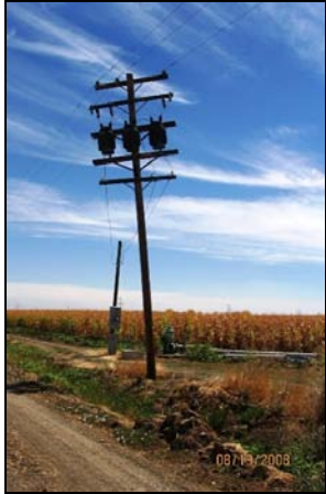
Photo 10: 3 pole-mounted transformers near Option D viewing east.
