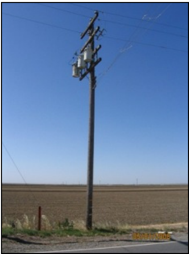
Photo 65: A pole mounted transformer located in the subject corridor.
