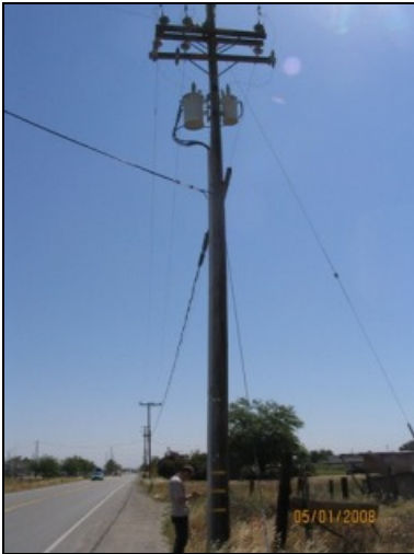
Photo 71: A pole mounted transformer located in the subject corridor.
