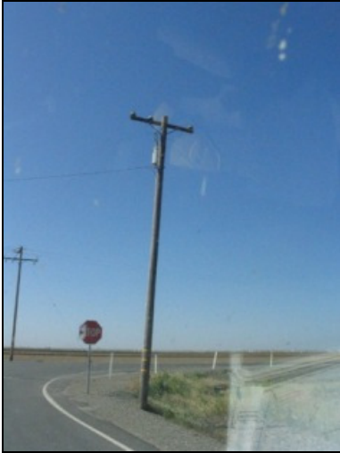
Photo 64: A pole mounted transformer located in the subject corridor.
