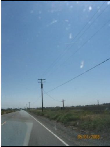
Photo 67: A pole mounted transformer located in the subject corridor.
