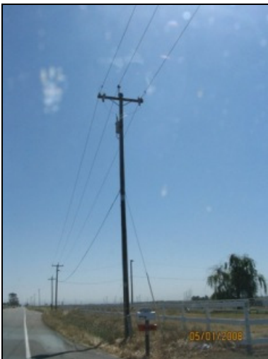
Photo 84: A pole mounted transformer located in the subject corridor.
