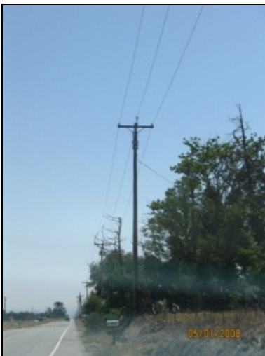
Photo 80: A pole mounted transformer located in the subject corridor.
