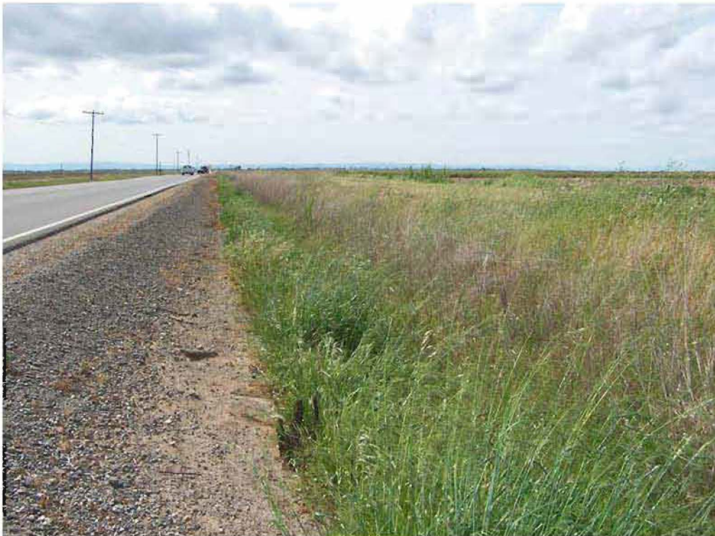
PG&E Line 407 East Project – OW135
