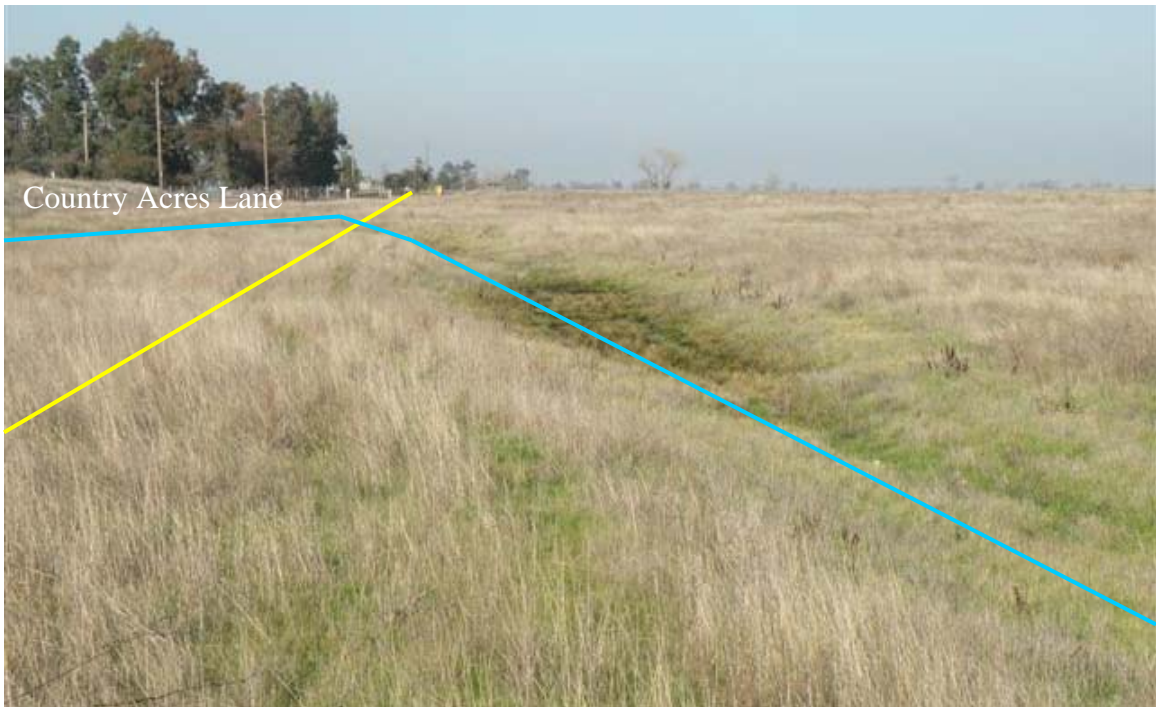
Drainage crossing the shared alignment along east side of Country Acres Lane 0.2 mile north of Base Line Road, facing north.
