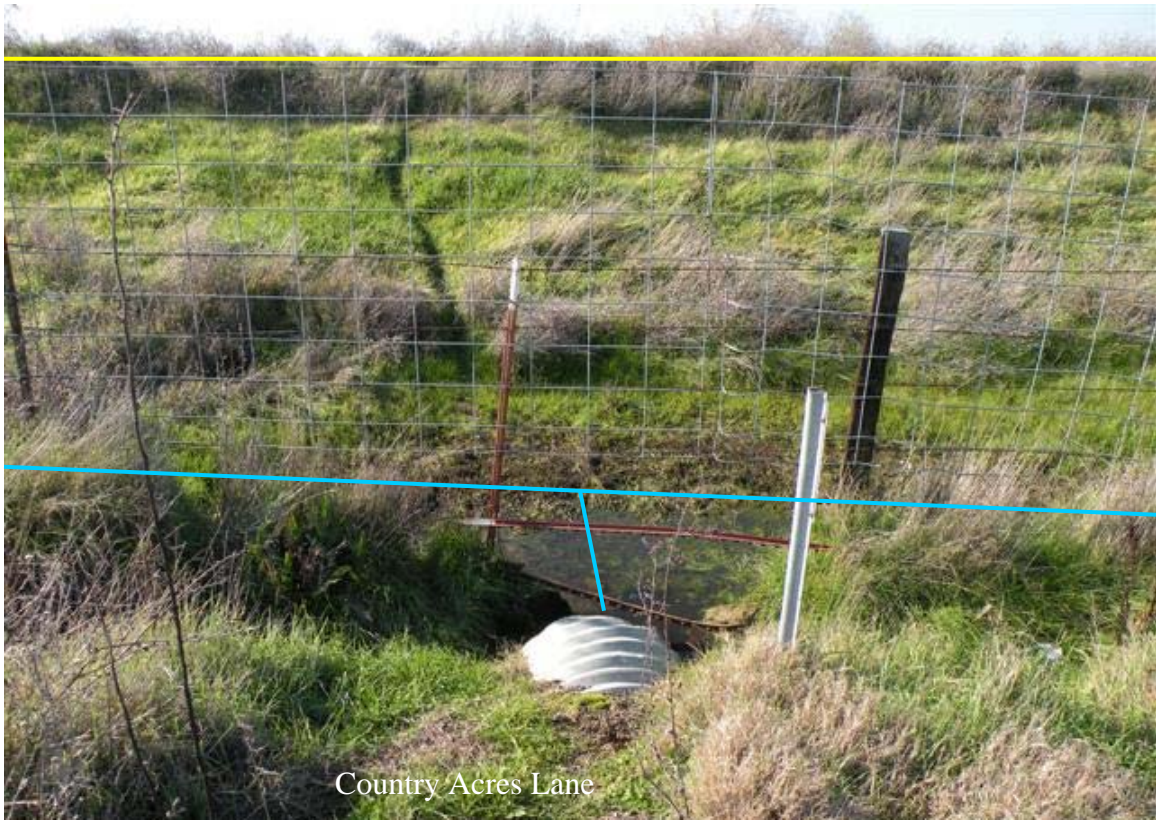
Roadside ditch east of the shared alignment along west side of Country Acres Lane 0.3 mile north of Base Line Road, facing west.
