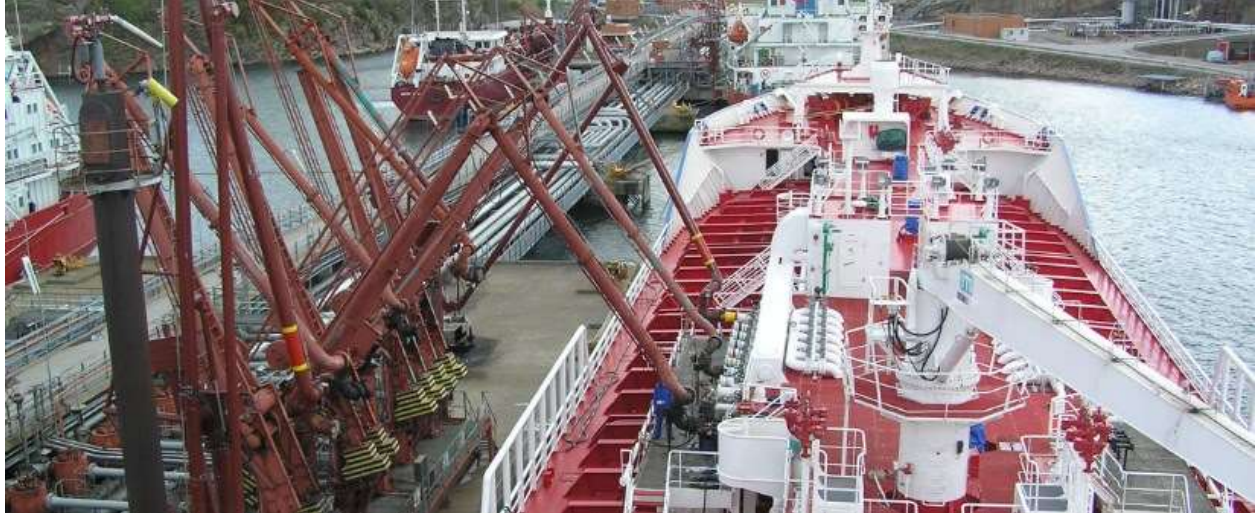
Figure 2 Brofjorden, Sweden marine terminal. Loading arms are similar in size to that needed for SA Recycling’s ballast water handling operations, but smaller than required for Stockton or El Segundo case studies. (source Marcus Bengtsson, wikicommons)
