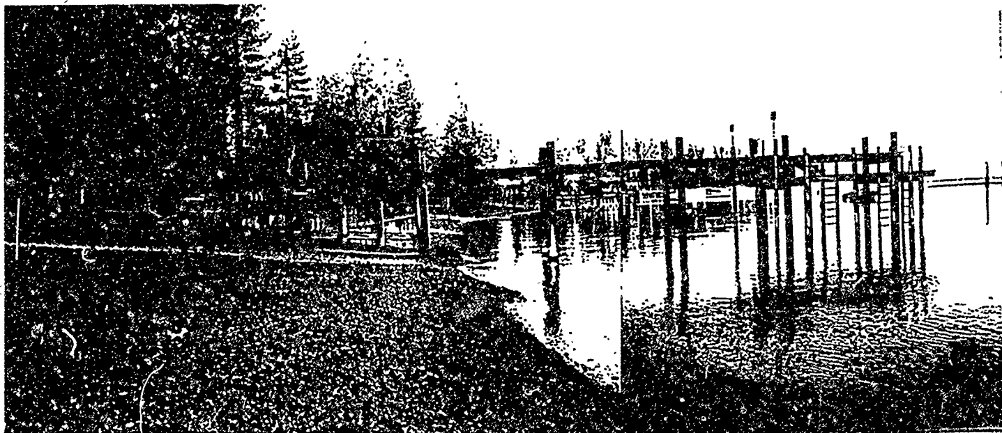
Most northerly pier - Northerly property line fence can be seen in the background
