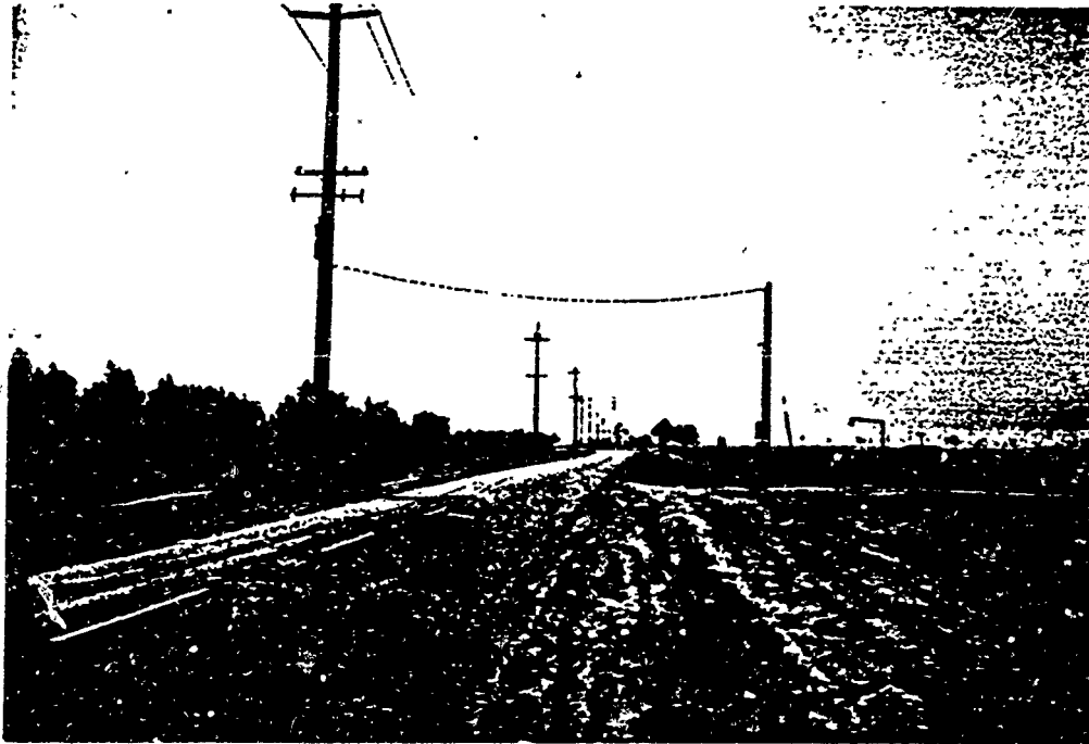
Looking south on Road 35 at the road crossing near Avenue 7. The line crosses at a bend in the road.
